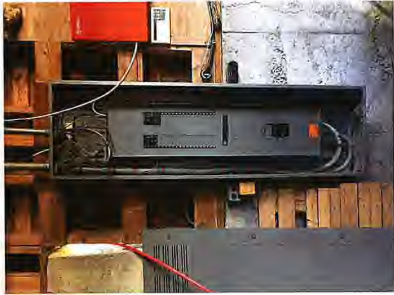
Electrical Safety Hazard – Exposed service panel
