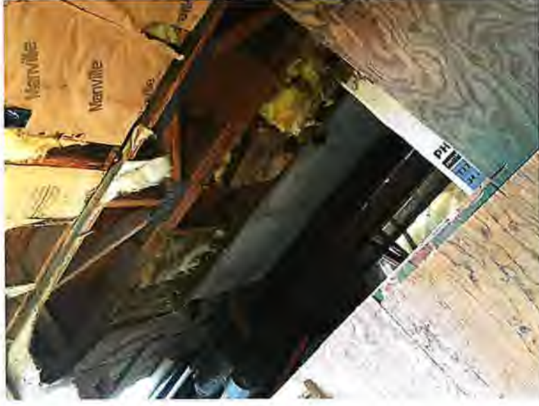
Opening in floor from main building level to basement – No stairs – Safety hazard
