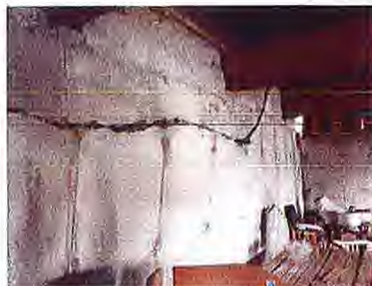
Horizontal Crack, Right end of Back Foundation Wall. Note Steel beams to be Supported
