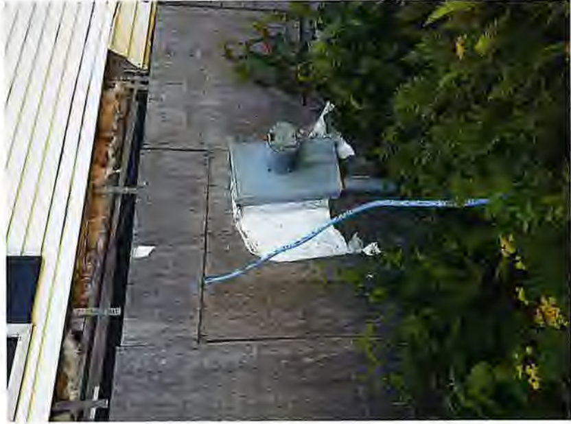
Gas line? entering building – Safety hazard
